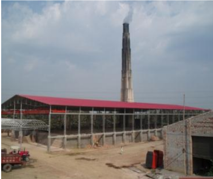
Zigzag Kiln (natural and forced draft)
